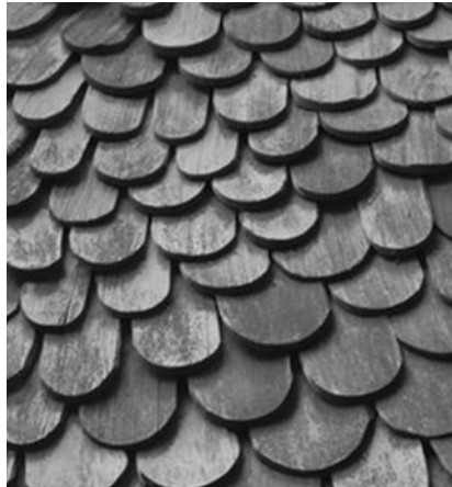
Charred Timber Shingles
